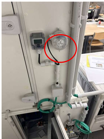
Figure 46 câblage final du pressostat
