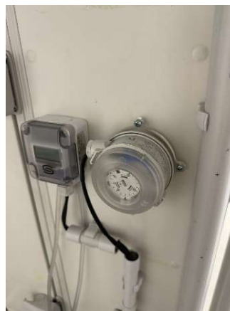
Figure 50 Pressostat fixé
